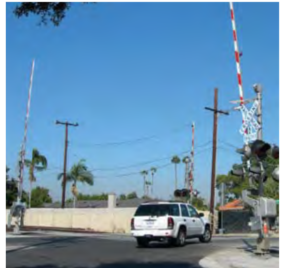
Grade crossing with quad gates
