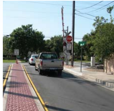
Grade crossing with raised center medians and safety gates
